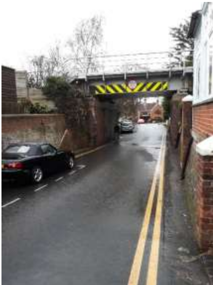
Looking North towards the bridge
