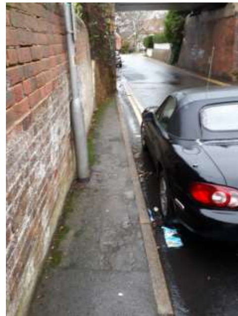
West side pavement 3
