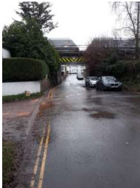
Looking South towards the bridge
